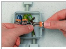
Termination:Insertstripped solid conductor until it hits backstop.
