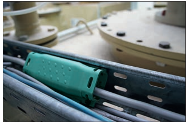
Relicon Relifix V gel cable joints.
