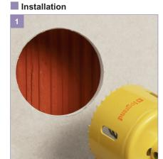
Hole cutter saw Ø67 Box Ø67 mm, more space for cabling
