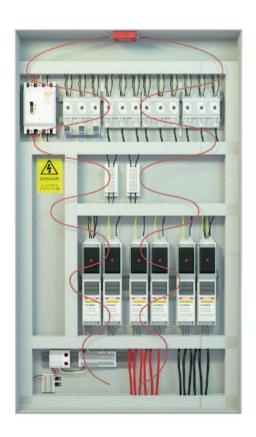
Make sure that the HDC cables are placed in the enclosure to optimise detection. Place the HDC cable close to every component that could be a potential fire hazard.
