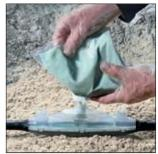
The filling nozzle in combination with the adapter makes filling the joint very easy and e†cient.
